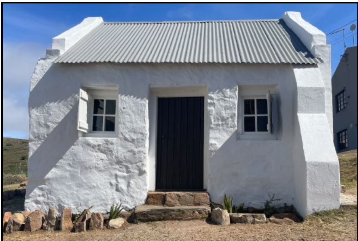
The completed restoration of Livingstone Cottage
